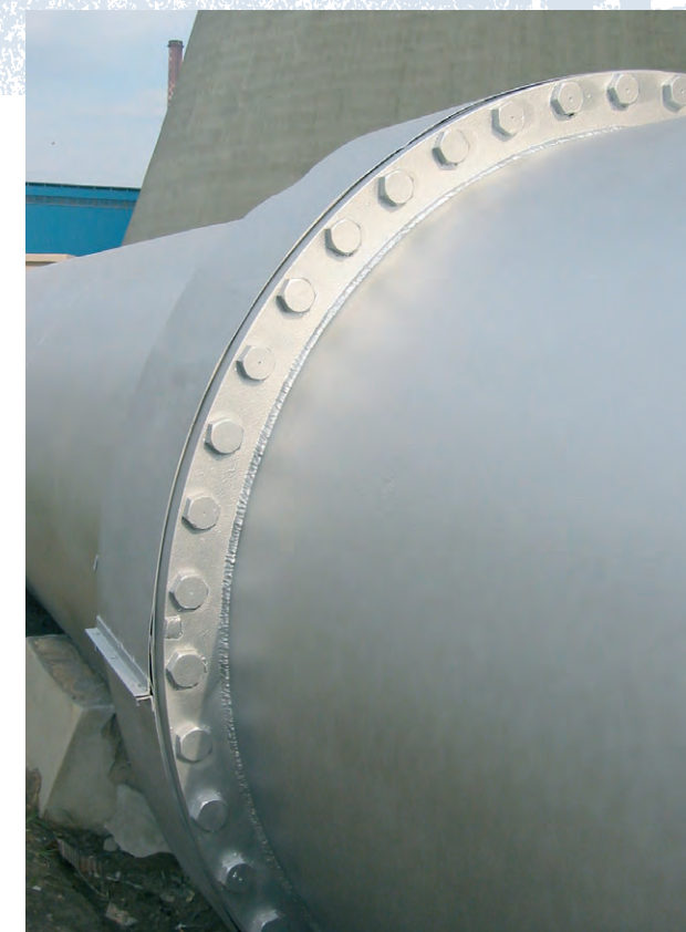
Potrubí po aplikaci antikorozního systému Piping after the application of the anti-corrosive system
