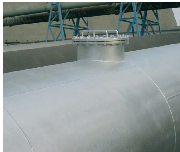
Potrubí po aplikaci antikorozního systému Piping after the application of the anti-corrosive system
